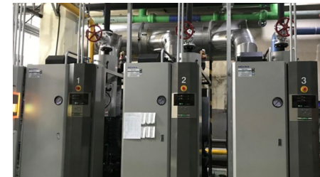
Installation of high-efficiency one-through boiler
