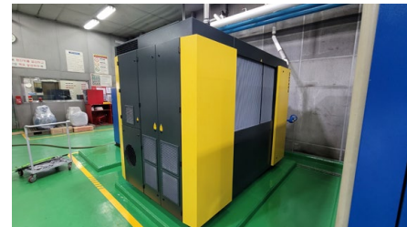
Installation of high-efficiency inverter-type air compressor
